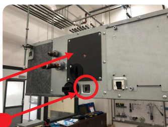
Drain pan inspection window
