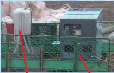
Extend fuel tank Generator
