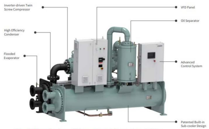
Hitachi Variable Speed Water-Cooled Screw Type Chiller WVY Series
