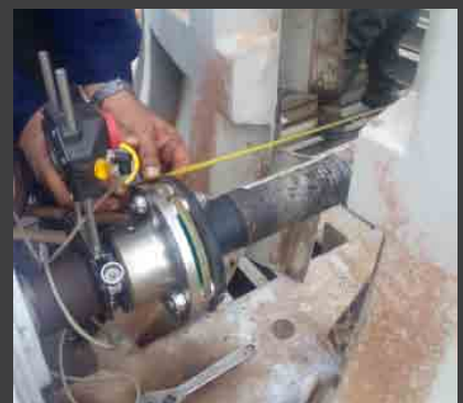
Alignment checking for gear reducer drive (shown above) and belt drive system.
