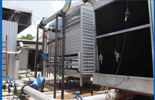
CTI testing of Genius cooling tower in progress.
