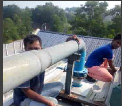
Changing of hot water basin for all brands of crossflow cooling tower
