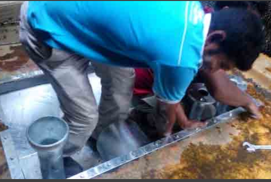
Changing of HDG steel water sump to new one
