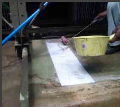
Lamination of FRP surface to repair leaks for all brands of cooling towers.
