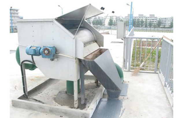
Drum filter installation diagram
