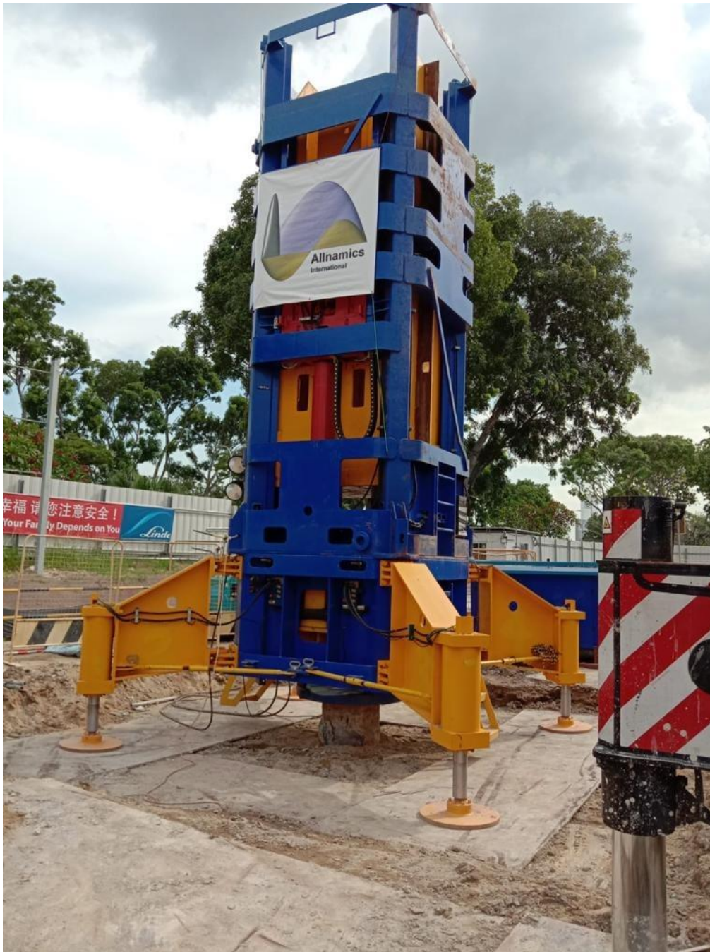
Photo: Dynamic Load Test at Construction Site
