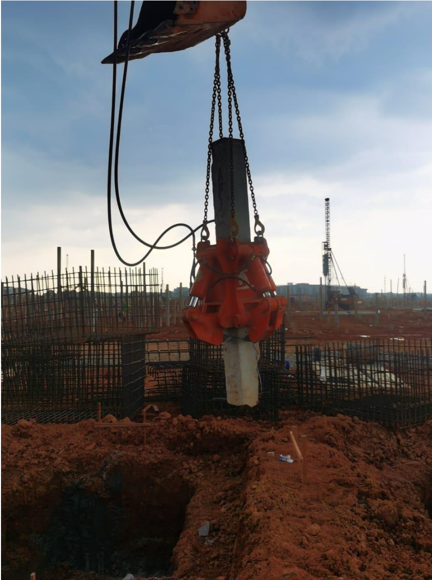
Photo: Pile Cutter working at construction Site
