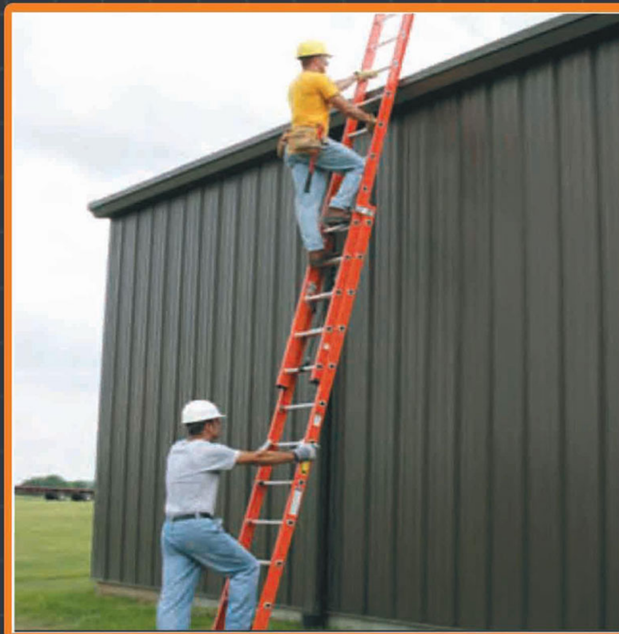
If possible, have another person hold the ladder when you are working on it.
