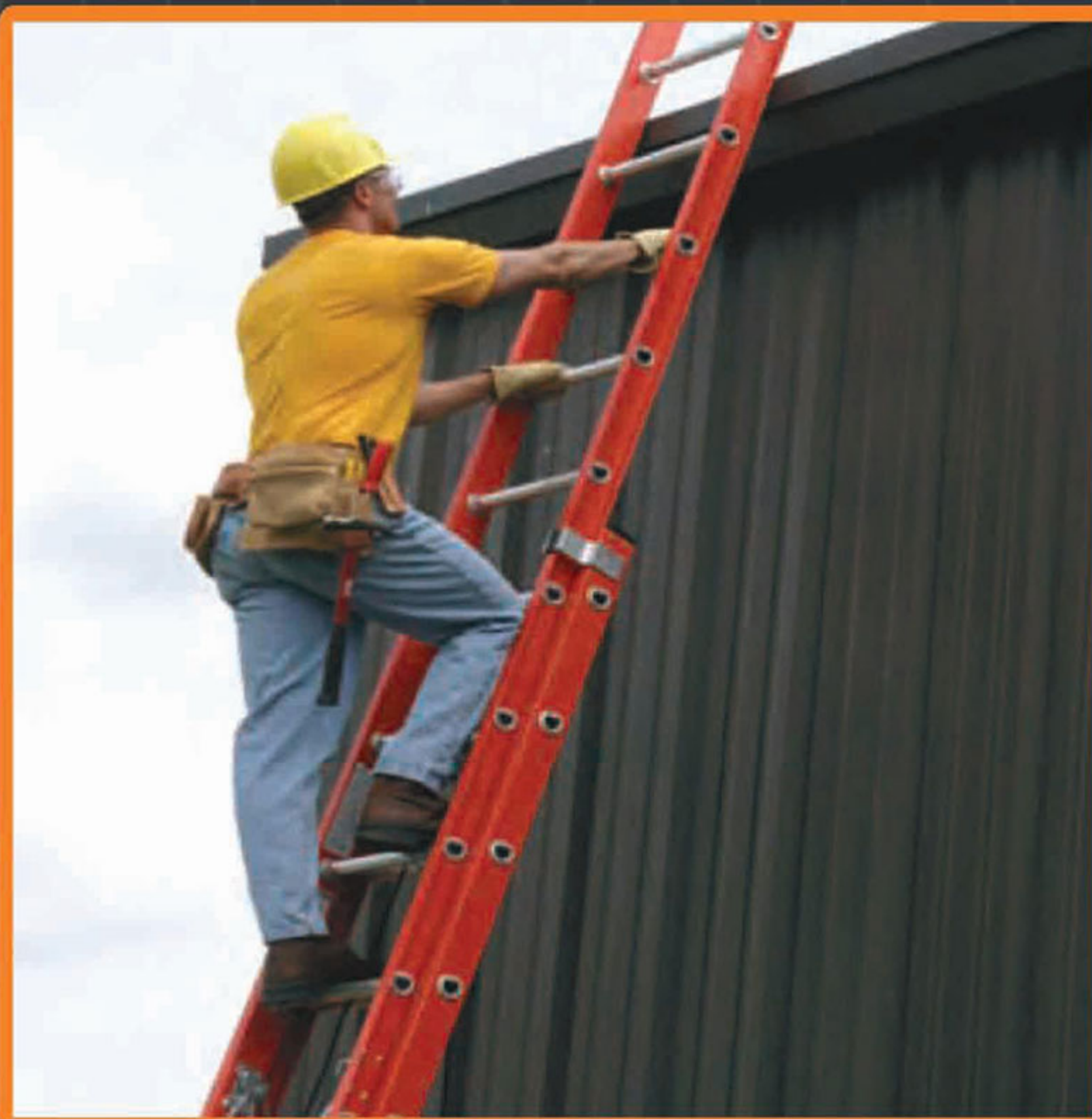
Climb facing the ladder. Center body between the rails. Maintain a firm grip.
