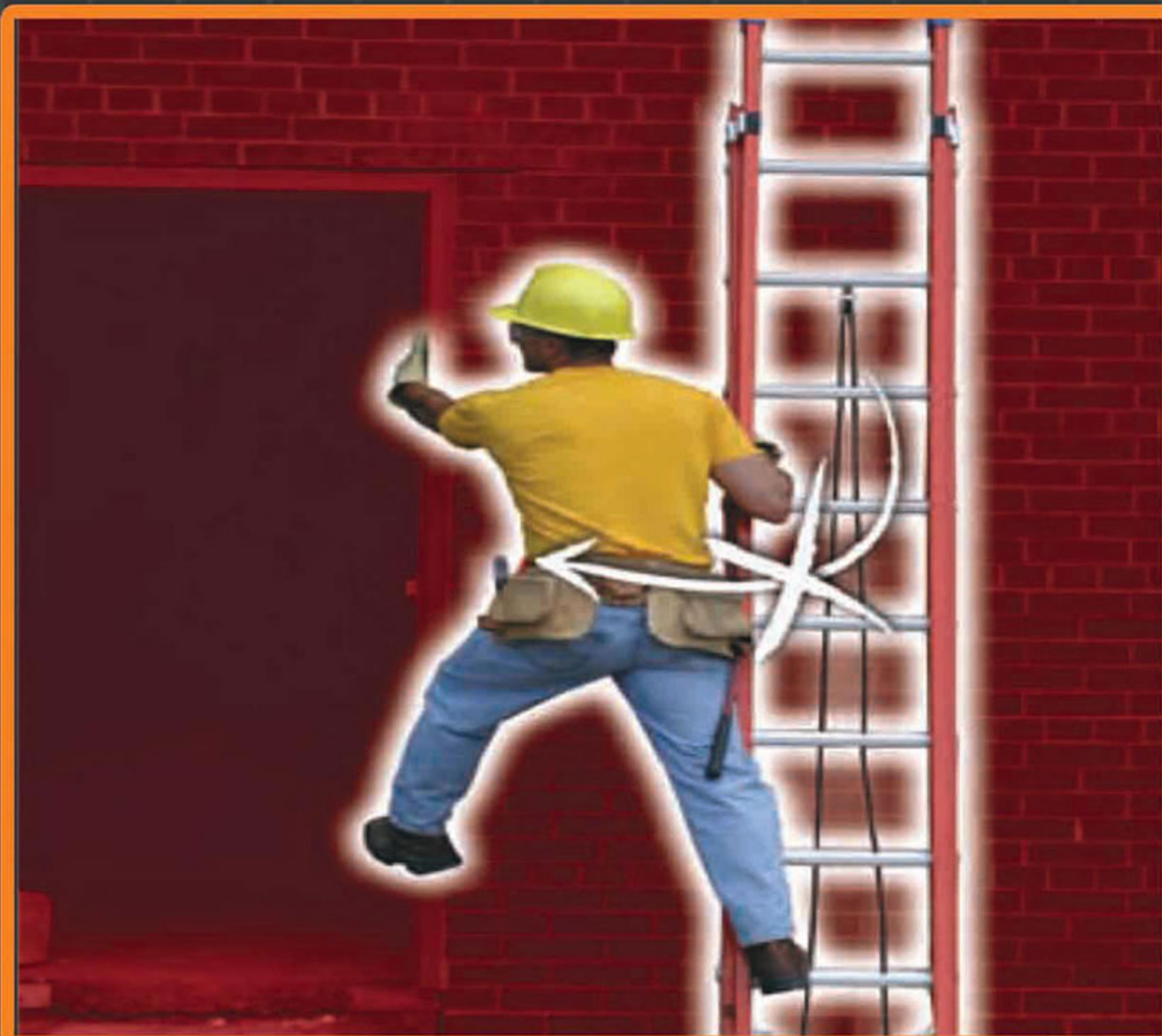
Do not climb on or off a ladder from the side. You could push the ladder away and fall.
