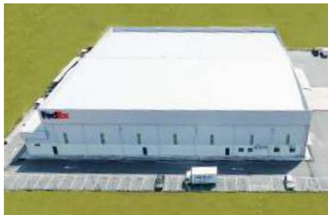
FedEx - FEDERAL EXPRESS SERVICES (M) SDN. BHD. Aluzinc AZ150 0.47mm TCT Clip Lock 672
