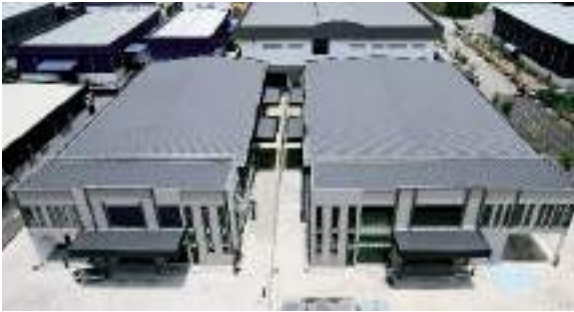
Realcolor Primero 0.47mm TCT Superior Rib PU Metal G26 in Volcanic Grey
