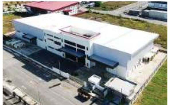
INDIUM CORPORATION (M) SDN. BHD. Aluzinc AZ150 0.47mm TCT High Rib Longrun
