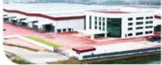
ASTINO METAL PENANG HEAD OFFICE
