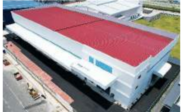
Realcolor Primero 0.47mm TCT High Rib PU Aluminium 25mm in Brick Red
