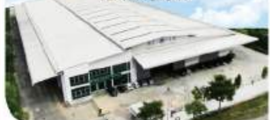
ASTINO COLOUR STEEL KL NEW FACTORY
