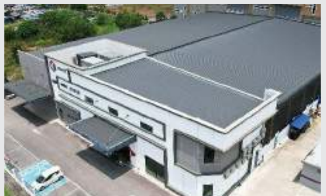
HUAYA PRECISION MANUFACTURING SDN BHD Realcolor Cahaya Plus 0.40mm TCT Superior Rib PU Metal 20mm in Volcanic Grey
