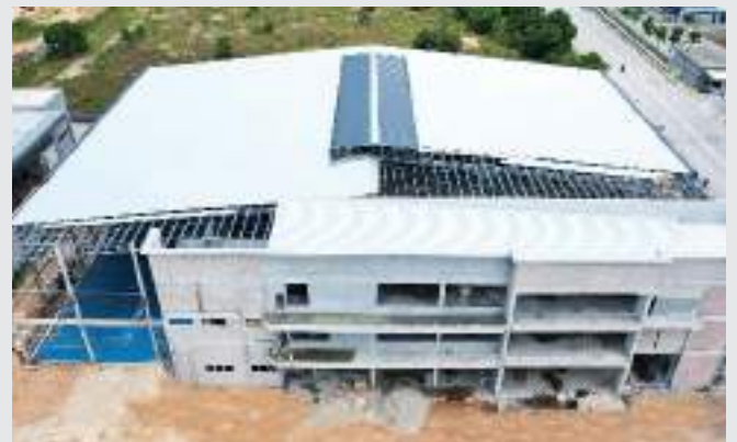
Aluzinc AZ150 0.47mm TCT Superior Rib Longrun
