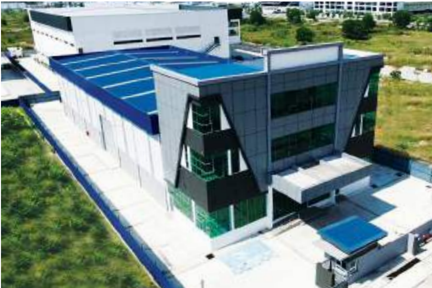
K.K. METAL PROCESSING SDN. BHD Realcolor Primero 0.47mm TCT High Rib PU Foam 25mm color in Fina Blue
