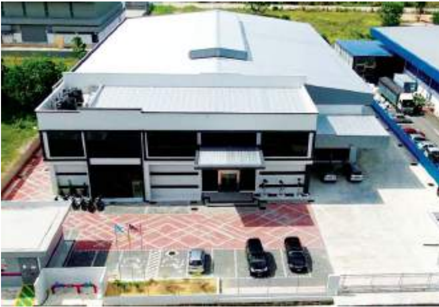
OSR MALAYSIA SDN. BHD. Aluzinc AZ150 0.47mm TCT High Rib PU Foam 25mm
