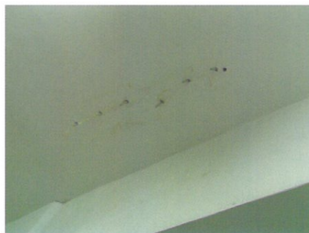
4. Curing and patching.
