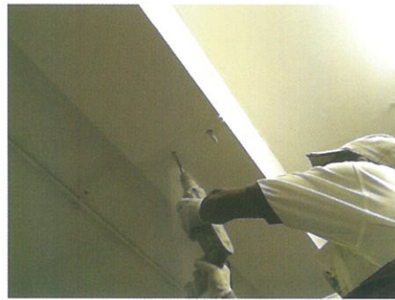
1. Drill injection holes.
