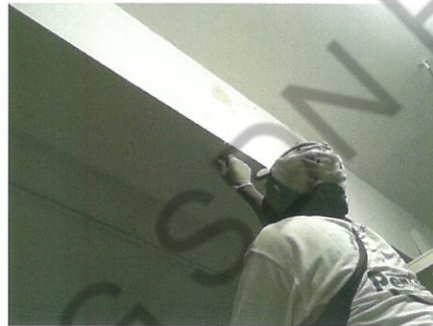
2. Insert injection packers.
