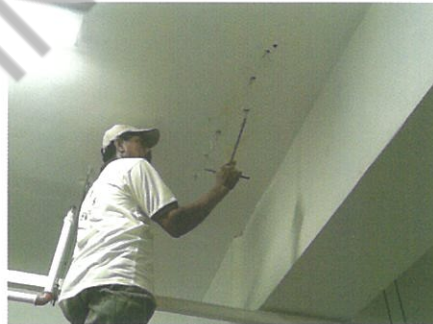
3. Crack injection.
