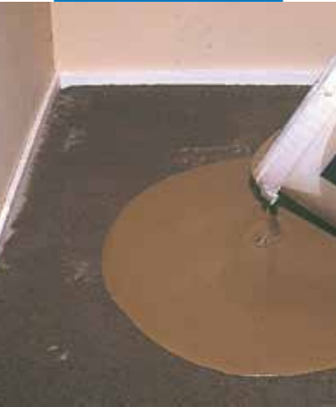
Applying the Novoplan 21 paste on the substrate
