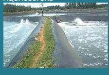
The applications of HDPE Geomembrane are widely trusted and used by Aquaculture facilities to contain and control quality of water from being contaminated. The different aquafarming such as:
