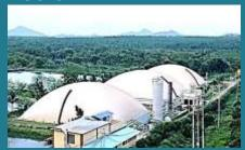
The HDPE Geomembrane covered anaerobic lagoon lining systems for industrial/domestic wastewaters. The applications such as:-
