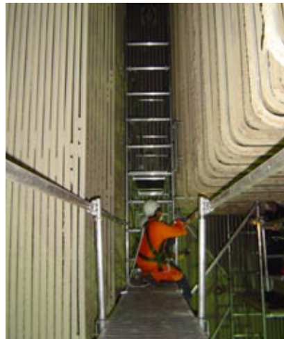
Above Left: Superheater Access Platform. Provides access for operators between superheater platforms
