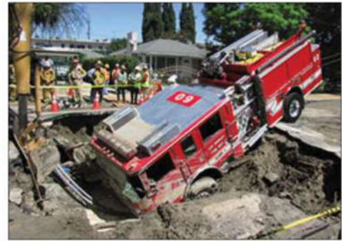
In Los Angeles, Calif., a fire engine drove over an unsupported layer of asphalt pavement and fell into a hole carved by a water main leak (Bardet et al, 2010).
