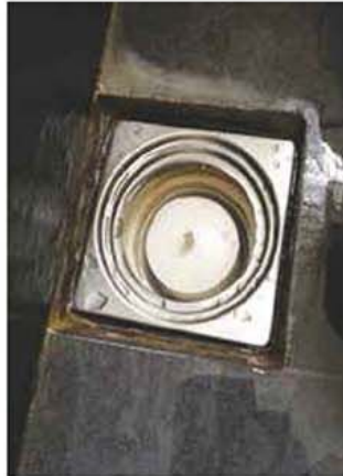
7 The trap (container and bell cap assembly) must always contain water to maintain the water seal integrity.
