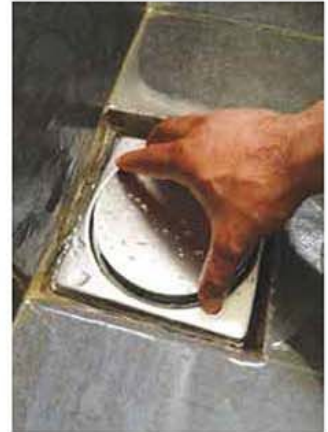
8 Return the grating or cover to its original position.
