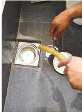
6 Return the container & bell cap assembly to its original position. (sit on the bottom of the trap) Fill up the container with clean water to create a water seal.
