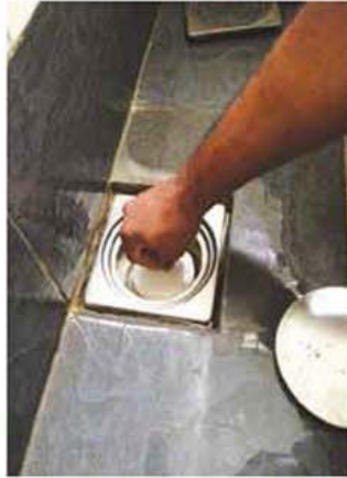
2 Remove the water seal trap (container & bell cap).
