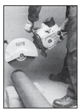
TCP pipes can be easily and quickly cut using either of the following methods. It should be ensured that the cut ends are square and any burrs removed. It should also be ensured that whatever cutting method is used, it complies with all relevant health and safety regulations and also with the safety guidelines from the cutting tool manufacturer's operating manual.
