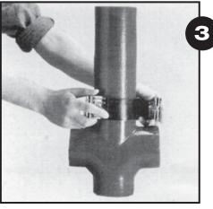
Wrap the TCP stainless steel collar around joint ensuring the gasket is within the collar.
