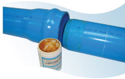
STEP 4 Apply lubricant to the spigot end and approximately mid-way back to the reference line.
