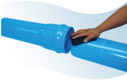
STEP 3 Clean the spigot end of the pipe as far back as the reference line.
