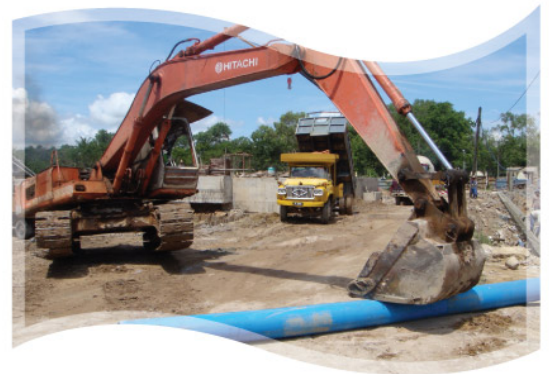
Load test conducted on M-PVC pipe by using a 20 tones excavator
