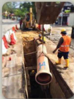
Installation of JPC Intan Socket Pipe at jobsite
