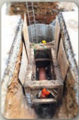
Installation of JPC Intan Socket Pipe at jobsite
