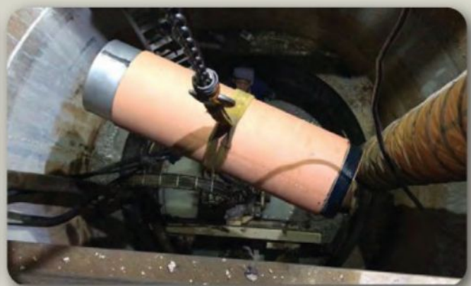
Installation of JPC Intan Jacking Pipe at jobsite
