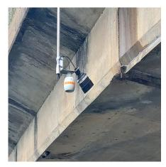
FarSight<sup>™</sup> and REFLECT<sup>™</sup> mounted with dBA0008 angled mounting bracket for areavelocity flow measurement
