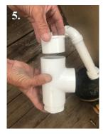
5.) If  $1\frac{1}{2}$ " pipe exists, cement the 2" to  $1\frac{1}{2}$ " reducer bushings into the tee (included with the R-40).
