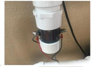
If the electrodes are worn out, they need to be replaced. Contact your dealer or visit <a href="https://www.ElectrodeWarehouse.com">www.ElectrodeWarehouse.com</a> or call Clearwater Enviro Tech for a replacement set. The entire chamber is replaced and a new set is screwed into the tee. Always use plenty of teflon tape around the threads to prevent leaking.
