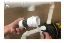
7.) Screw the electrode into the downward facing tee. Tighten only by hand, do not use any tools to perform this step.
