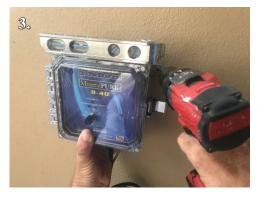
**3.)** Mount the control box to the wall allowing for the power cable to reach the source of power and the electrode wire to reach the electrode chamber. Use proper anchors and screws to mount. (Not provided)
