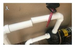
3.) Using a hacksaw or backsaw, cut a 3" gap in the section of pipe if 2" pipe exists, or cut out a 4" gap if a  $1\frac{1}{2}$ " pipe exists.
