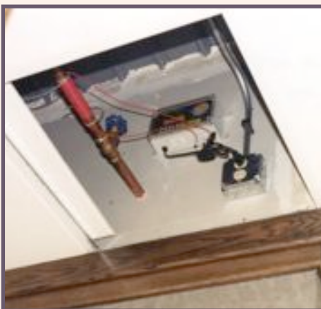
This new Arby's store had ScaleBlaster's installation pre-planned and was mounted in the ceiling and hidden by a dropped ceiling pad.
