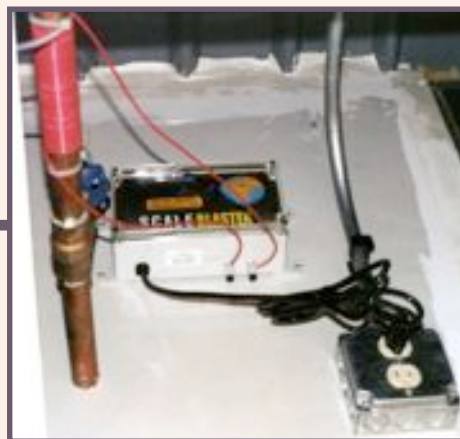
This new Arby's store had ScaleBlaster's installation pre-planned and was mounted in the ceiling and hidden by a dropped ceiling pad.
