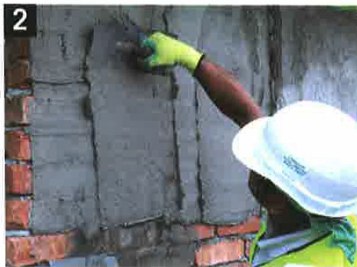
2 Plaster first layer (10-15mm thickness)
