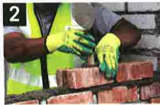
Lay bricks and secure with trowel's handle
