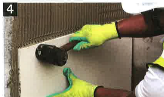
4 Secure the tile with rubber mallet
