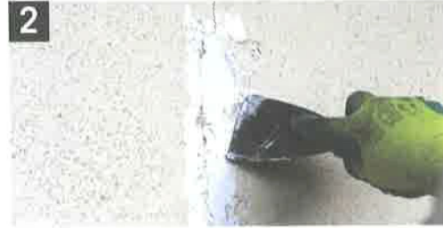
2 Fill the formed channel with LiquidRepair 1000
