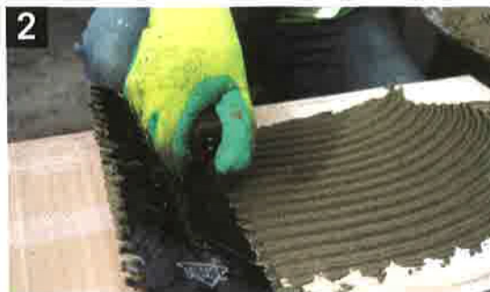
2 For tiles size ≥300mm x 300mm, apply a thin layer at the back of tiles
