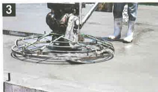
3 Further smoothing with steel trowel / power-float
