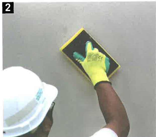
Surface can be sponged to obtain consistent semi-smooth finishes
