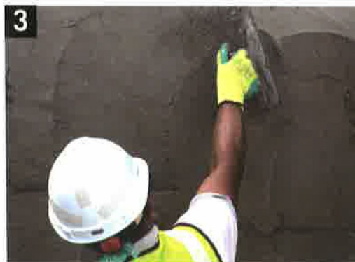
3 Plaster second layer (5-10mm)
