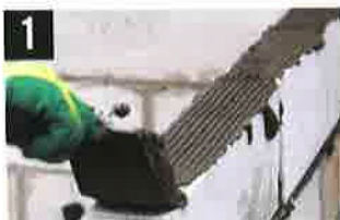
Apply mortar adhesive on block units with notched trowel
