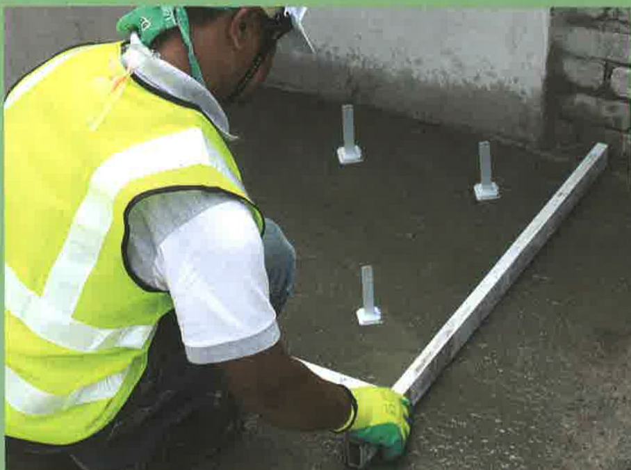
Set out level pegs/indicator at regular interval
