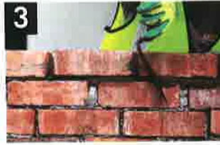
Remove excessive mortar
