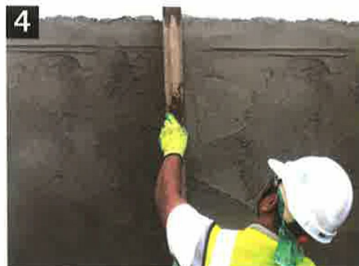
4 Level the surface with long wood float
