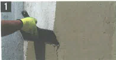
1 Level surface with base coat (2-5mm)
