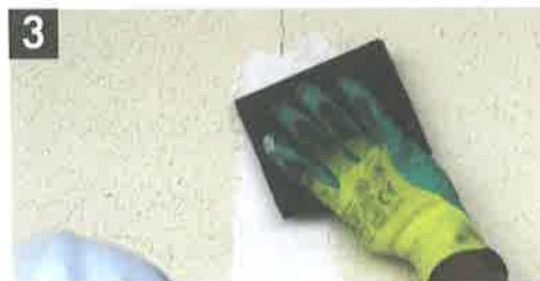
3 Smoothen the surface with sandpaper after filler has set
