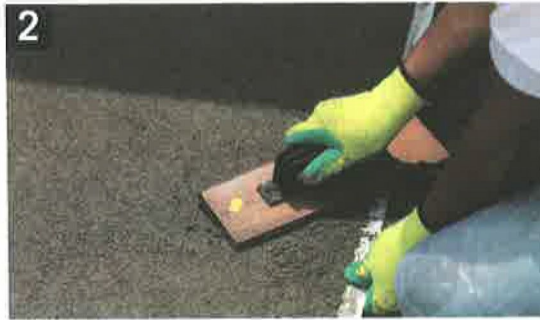
2 Apply Floor Screed 383 and level with wood trowel
