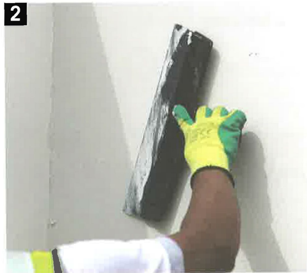
Smoothen surface with top coat (1-2mm)
