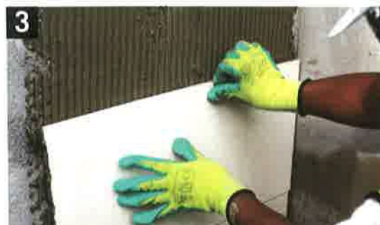
3 Lay tile onto the wall / floor substrate with light adjustment
