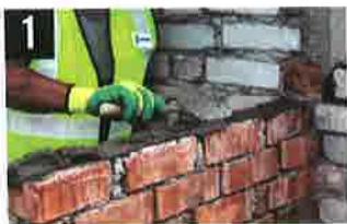
Spread mortar on bricks
