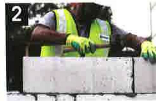
Lay block and secure with rubber mallet
