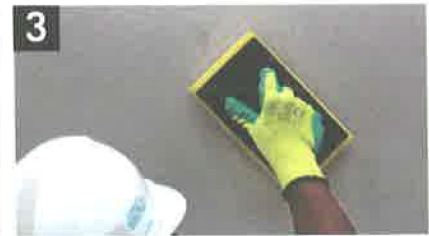
3 Surface can be sponged to get consistent semi-smooth finish wall
