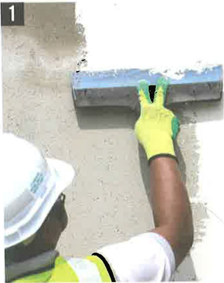
Level surface with base coat (2-5mm)
