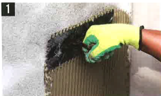
1 Apply adhesive uniformly with appropriate notched trowel onto the wall / floor substrate
