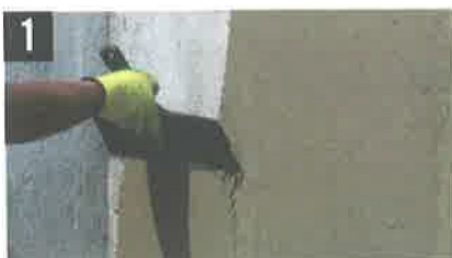
1 Level surface with base coat (2-5mm)
