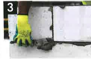
Remove excessive adhesive mortar
