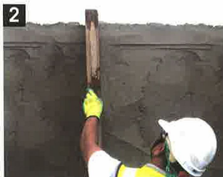
2 Level the surface with long wood float
