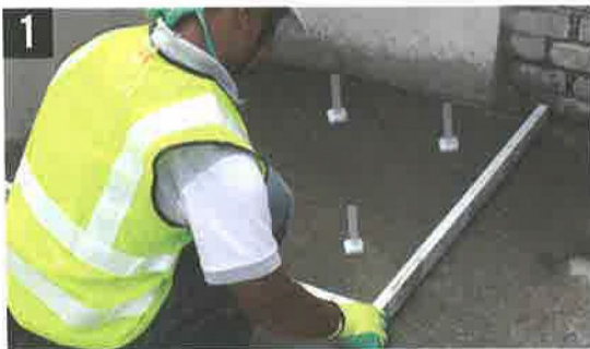
1 Set out level pegs/indicator at regular interval
