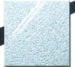
Breaking pattern of tempered safety glass
