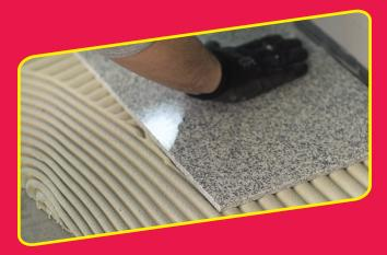
Fix tiles onto the adhesive bed, followed by a slight twisting action to secure contact. Touch the adhesive bed periodically to check for skin-over.
