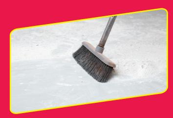
All surfaces must be clean, sound, and free from any laitance, oil, grease, and any contaminants.
