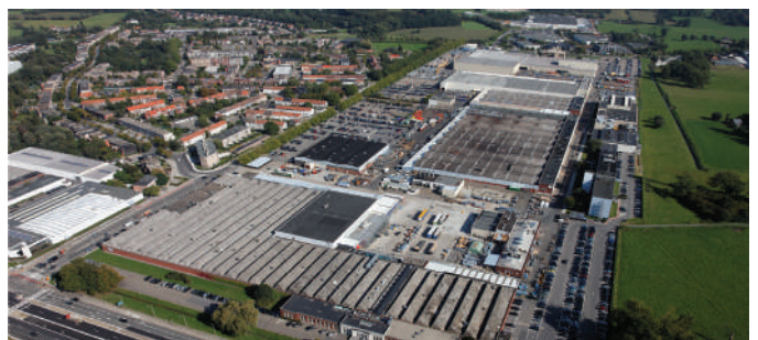
Oil and water injected screw compressors plant: Belgium
