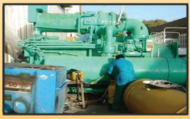
**Above:** Chillers containing **4000 lbs** of R134a being recovered with a **G5Twin** in the sweltering heat of Saudi Arabia. What once took a week now takes **only 18 hours** with the **Speed and Reliability** of the G5Twin
