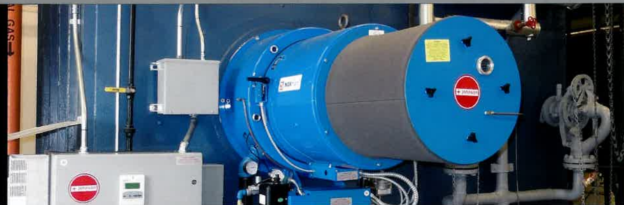
Low NOx mesh burner
