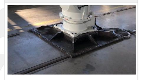
Installation steps of station plate/I-shaped riser and ground
