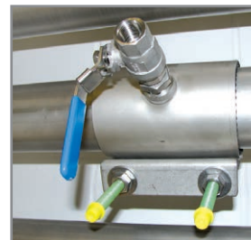
B Spot drilling collars
