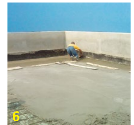
6 Cover with cement screed after 2nd layer.
