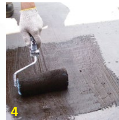
4 Apply directly to construction surface by using brush, roller or spray method.
