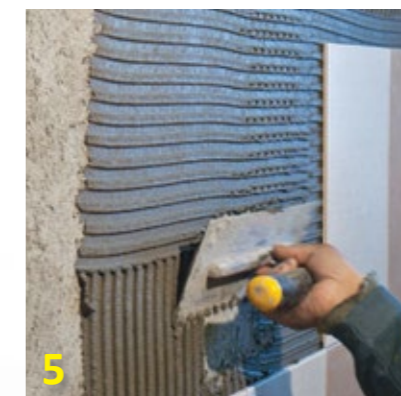
5 Apply directly to construction surface by using cement knife.
