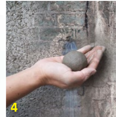
4 Put onto leaking area.
