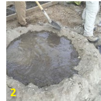
2 Add 15 litres clean water to mix container.
