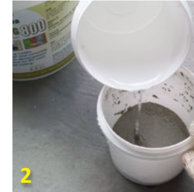
2 Add 1 litre water : 4kg powder to mix container.
