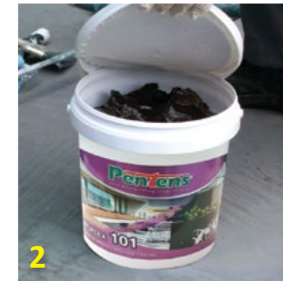
2 Open the cover of BITUFLEX 101. Add 0.7kg clean water to mix container.
