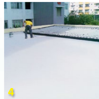
4 Apply second layer after 4 hours.
