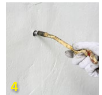
4 Fix the grouting hose into the packers and start grouting.
