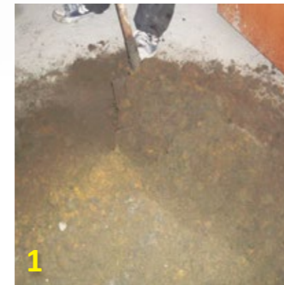
1 Mix together 50 kg cement & 150 kg sand.
