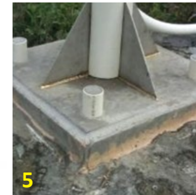
5 Remove the pile wood.
