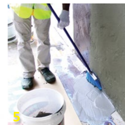
5 Apply directly to construction surface by using brush, roller or spray method.
