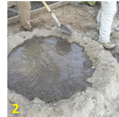
2 Add 15 litres clean water to mix container.
