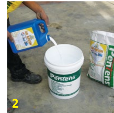
2 Add resin (part A) to an empty pail.
