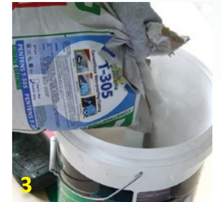
3 Add powder (part B) to mix container.
