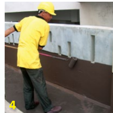
4 Apply directly to construction surface by using brush, roller or spray method.
