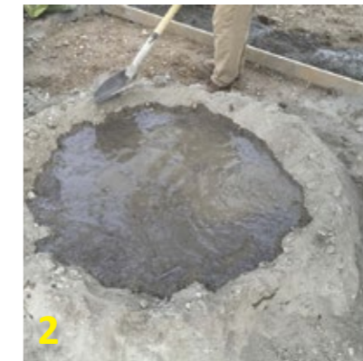
2 Add 15 litres clean water to mix container.
