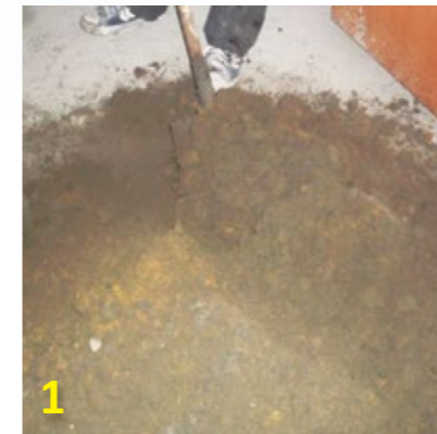
1 Mix together 50 kg cement & 150 kg sand.
