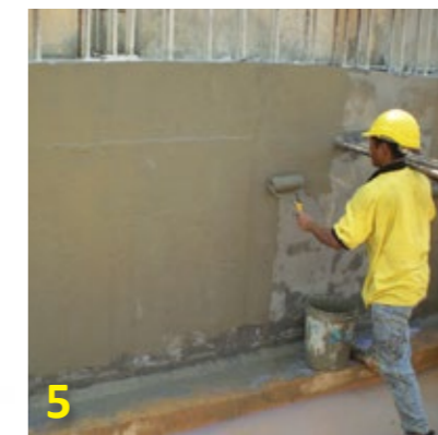
5 Apply directly to construction surface by using brush, roller or spray method.
