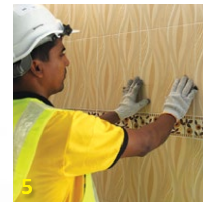
5 Tiles completely apply on wall area.
