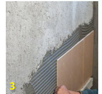
3 Laying the tiles on the wall or floor area.
