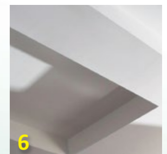
6 Remove the packer and cover with paint.
