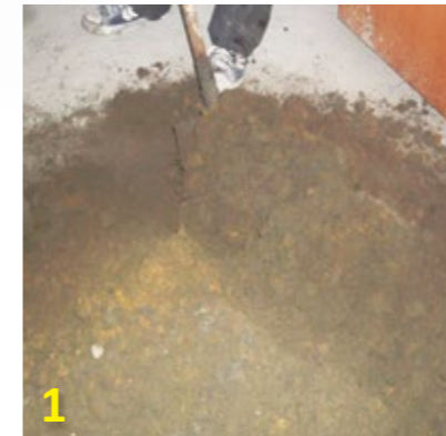
1 Mix together 50 kg cement & 150 kg sand.
