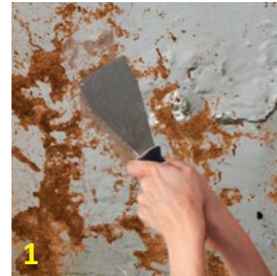
1 Remove debris from the structure completely.
