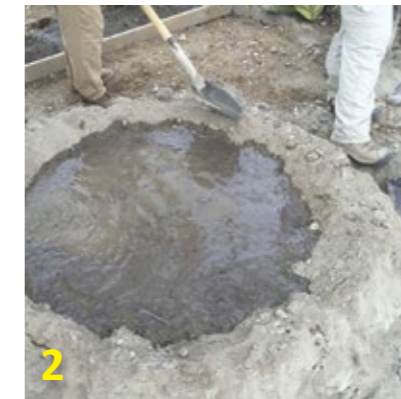
2 Add 15 litres clean water to mix container.
