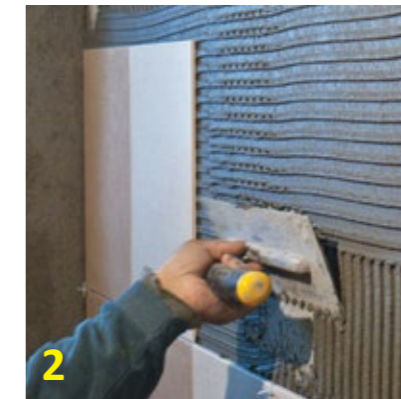
2 Apply the adhesive layer on the wall.
