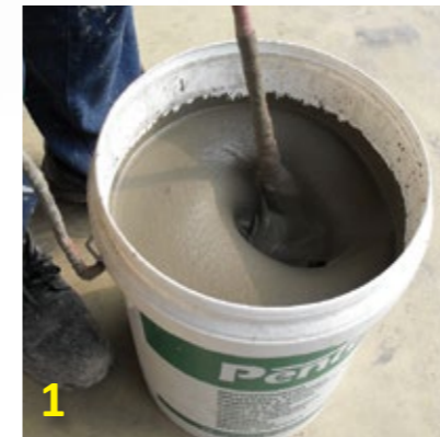
1 Add 6 - 6.5 litres clean water & TA-BOND 888, mix thoroughly.
