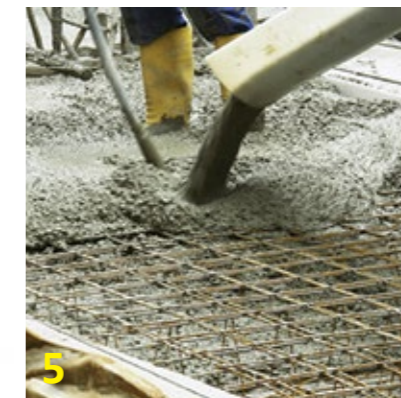
5 Then evenly pour the material on the construction surface.
