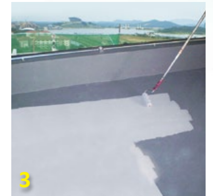
3 Apply directly to construction surface by using brush, roller or spray method.
