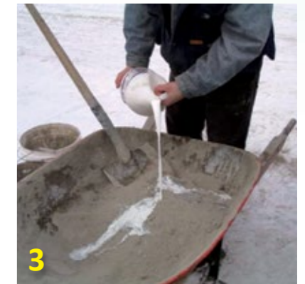
3 Add 4 litres Pentens Waterproof in cement sand.
