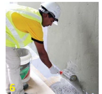
6 Apply directly to construction surface by using brush or roller.
