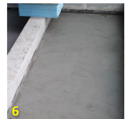
6 After 2 layers cover with cement render.
