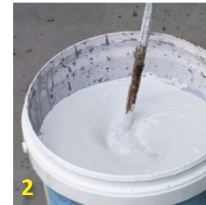
2 Open & mix thoroughly. (Can add 10% clean water to mix container)
