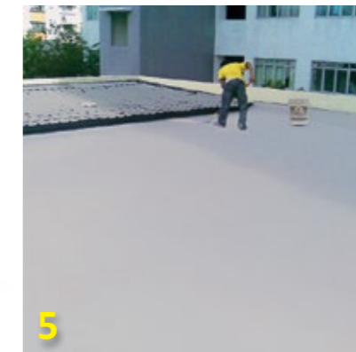
5 Apply second layer after 4 hours.
