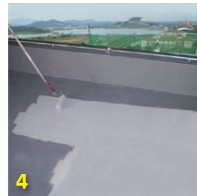
4 Apply directly to construction surface by using roller.
