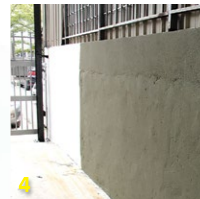
4 Finish with cement screed or tile.
