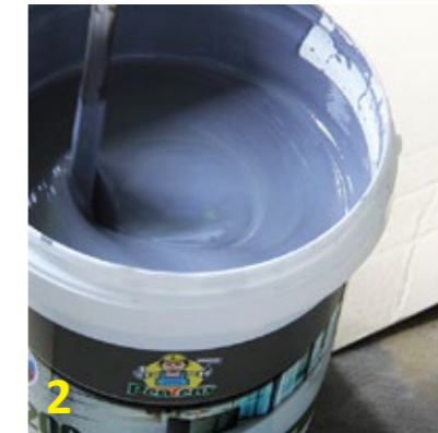
2 Open the cover of FLESEAL T-200 and mix thoroughly. (Can add 0.3kg clean water to mix container.)
