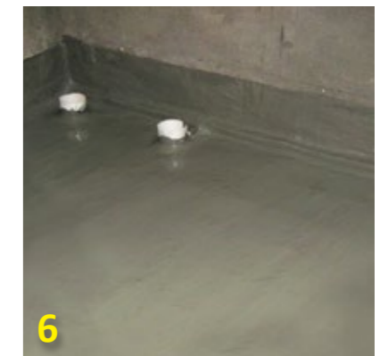
6 After 2 layers cover with cement render.
