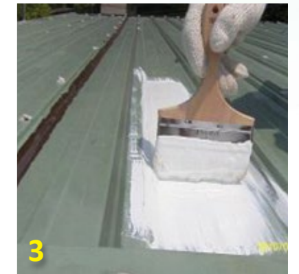
3 Apply directly to construction surface by using brush, roller or spray method.
