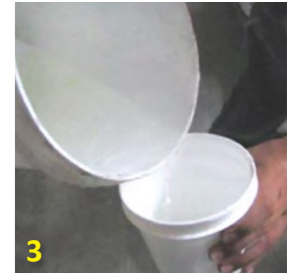
3 Add 1 litre water: 3kg powder to mix container.
