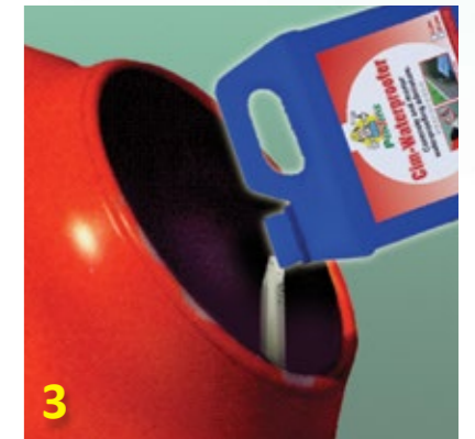
3 Add 4 litres Pentens CIM-Waterproofer in cement sand.
