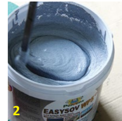
2 Open Pentens EasySov WP5+ and mix thoroughly. (Can add 0.3kg clean water to mix container)
