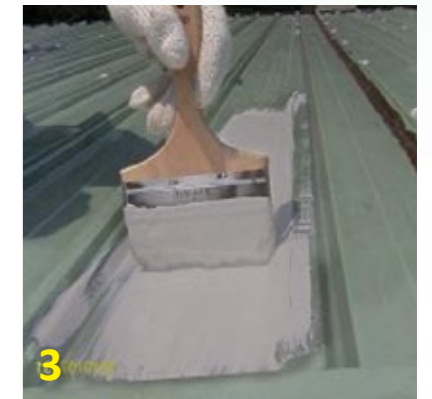
3 Apply directly to construction surface by using brush or spray.
