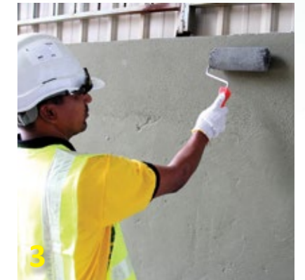
3 Apply directly to construction surface by using brush, roller or spray method.
