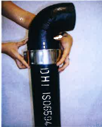
3. Insert the fittings spigot into the rubber gasket.
