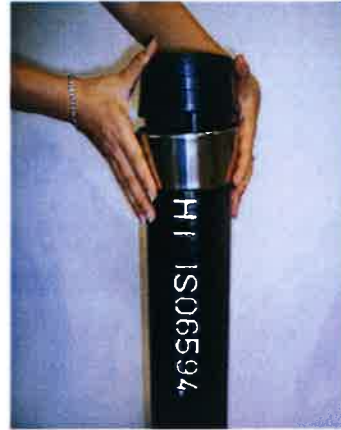
2. Put the rubber gasket onto the spigot of the pipe.
