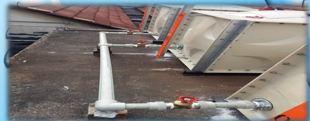
PLUMBING WORKS & PIPING SYSTEM
