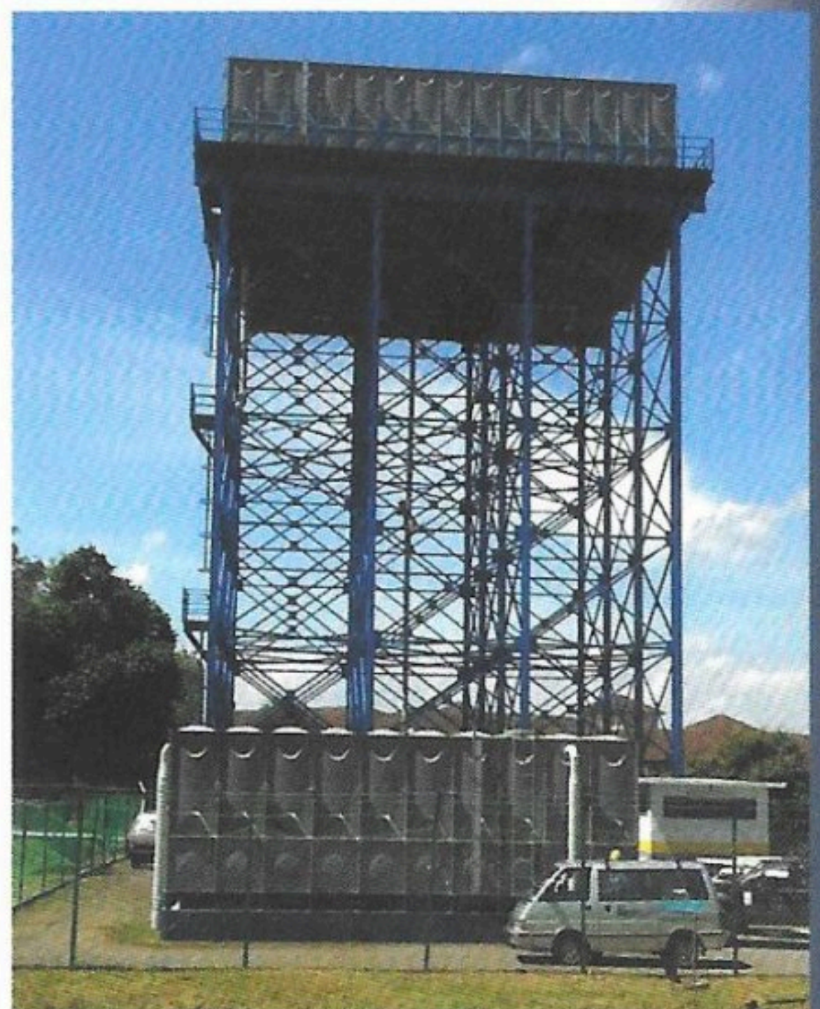
Installation of FRP Tank
