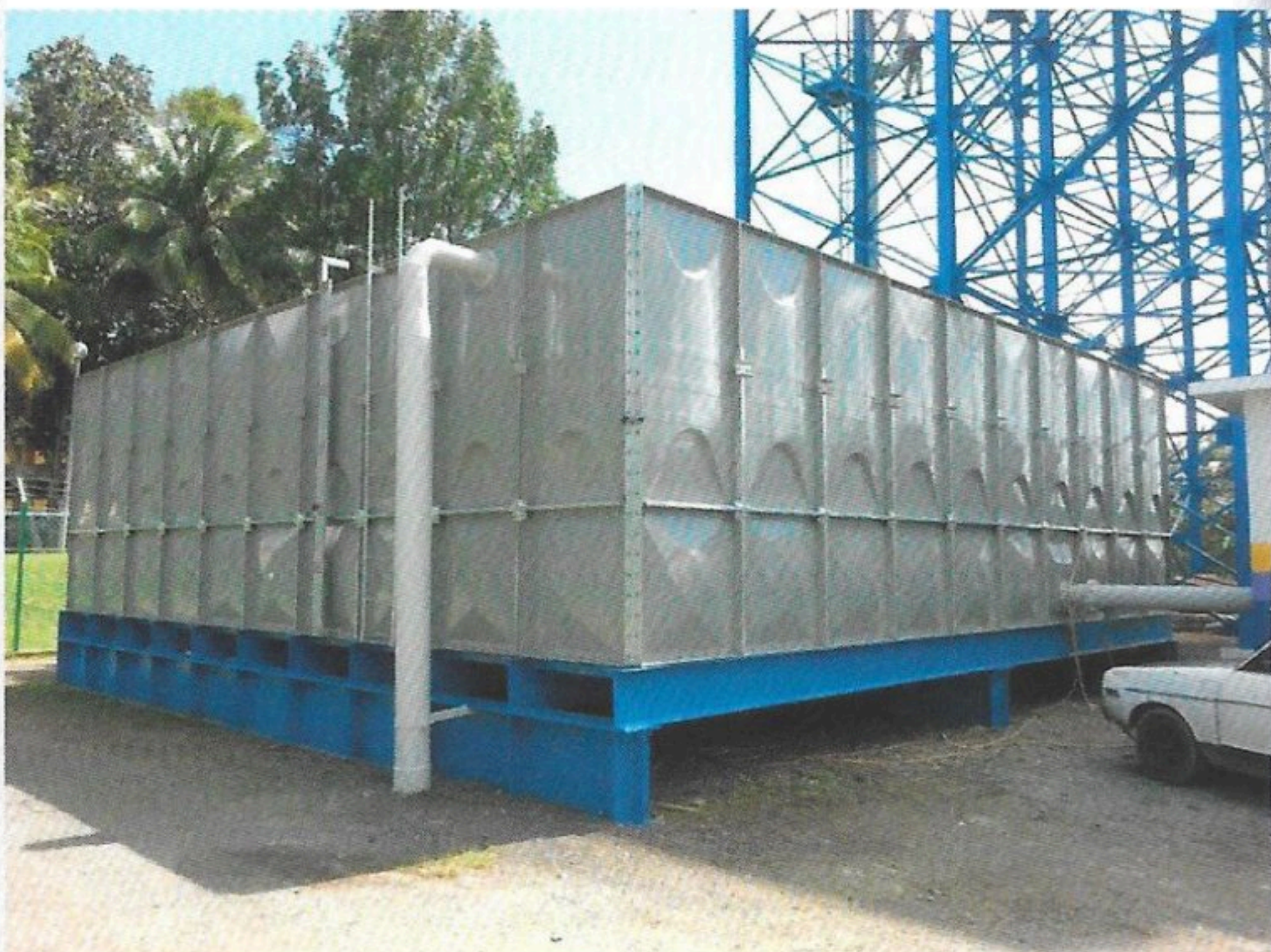
Installation of FRP TANK
