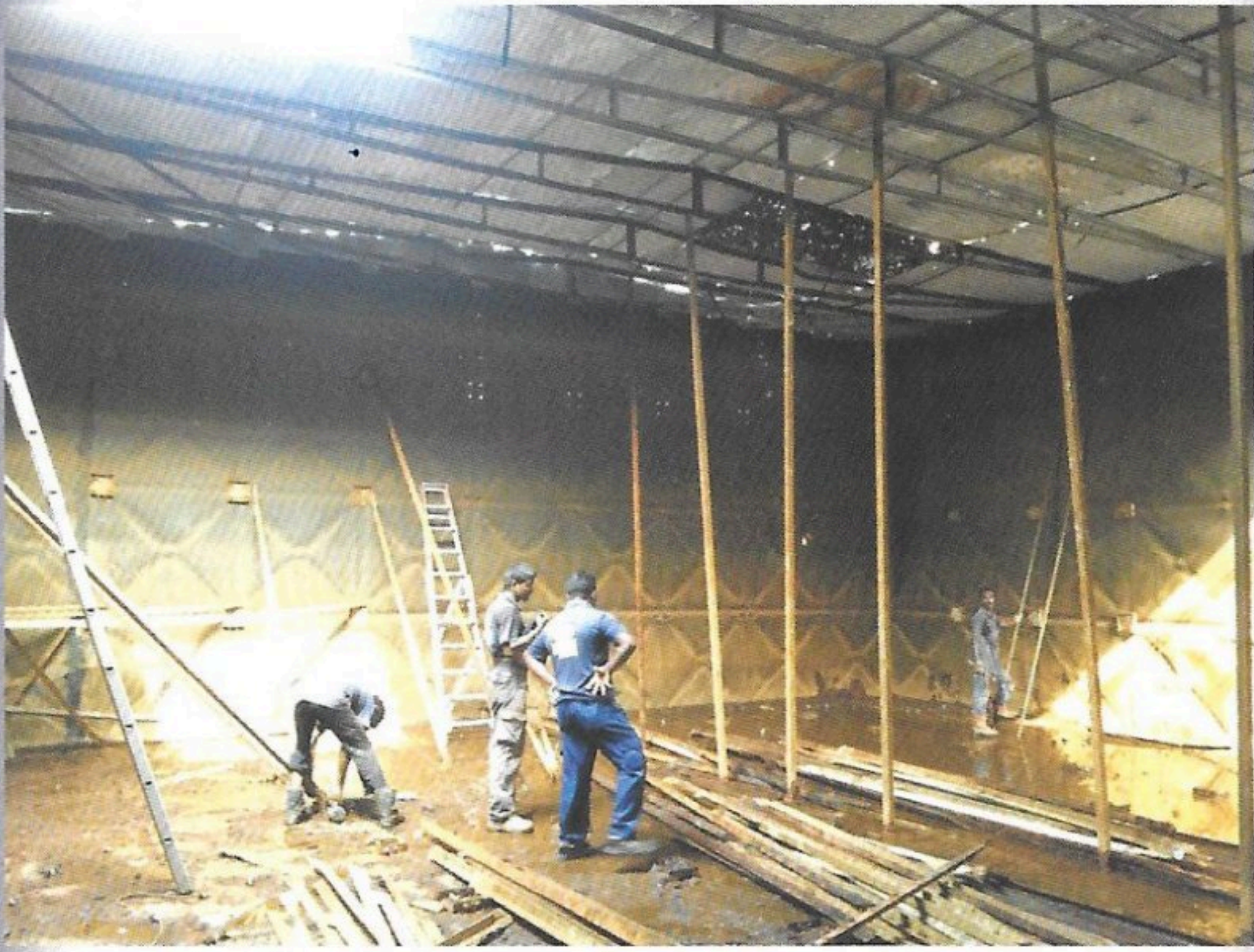
Refurbishment of water tank
