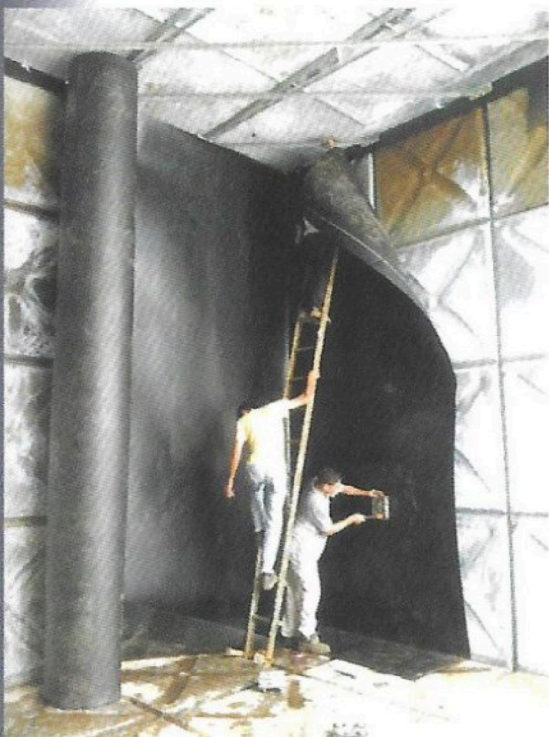
HDPE Lining Installation
