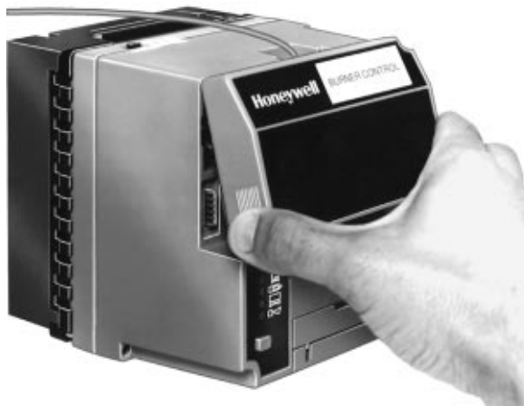
Fig. 11. Extension Cable Assembly mounting.
