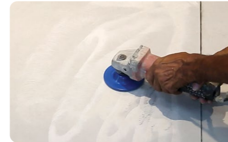
STEP 1 : GRINDING
