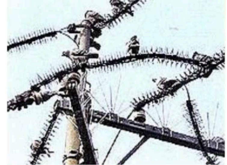
Failure of Needle Hill 3
