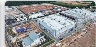
PDG TNB Substation Kidex, Johor
