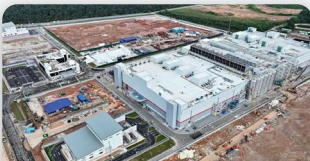
PDG JH1 Data Center Phase 1 KIDEX, Johor
