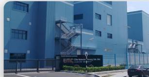
Elite Material TNB Substation Penang
