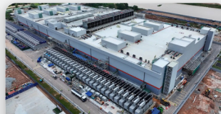
PDG JH1 Data Center Phase 4 KIDEX, Johor
