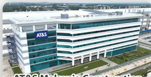
AT&S Malaysia Construction Project Phase 1 Kulim
