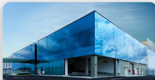
IPDC Data Center Johor
