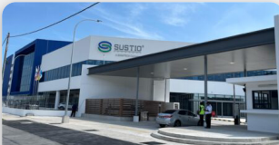
Sustio TNB Substation Batu Kawan
